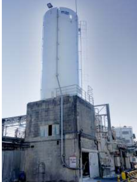
Silo through a concrete ceiling:
