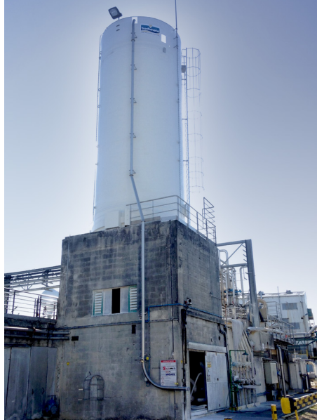
Silo through a concrete ceiling:
