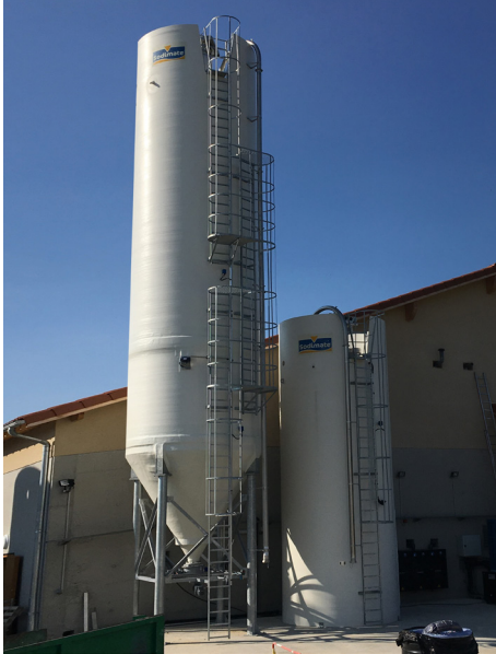
Legged and Skirted silos:
