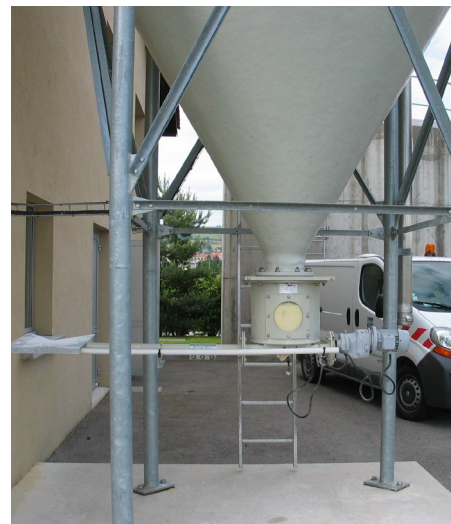
► Application case in water treatment for lime feeding (doc. SODIMATE)
