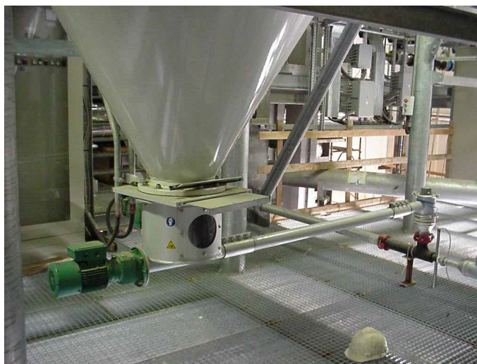
► Example of an industrial installation of a bridge breaker-feeder (doc. SODIMATE)
