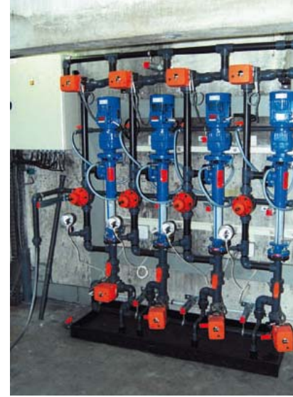
To comply with the aforementioned specifications, Sodimate selected four reliable, vertically mounted progressive cavity pumps for PAC slurry feeding.
